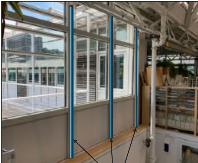
Hot Water Pipes
