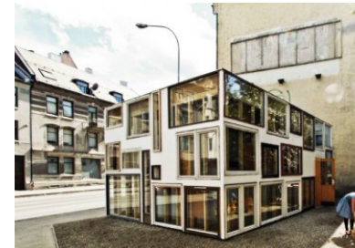
recycled architecture - rake
