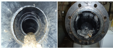
Figure 1 Image of deposits found in the flow meter (inlet) and pumps
