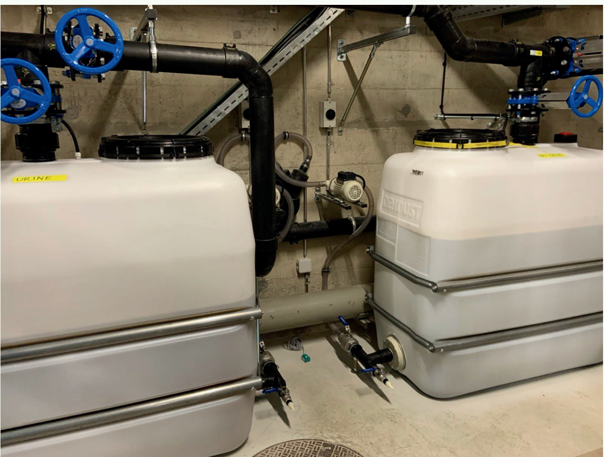
Two tanks (urine and GW) under two sanitary blocks at the CE
