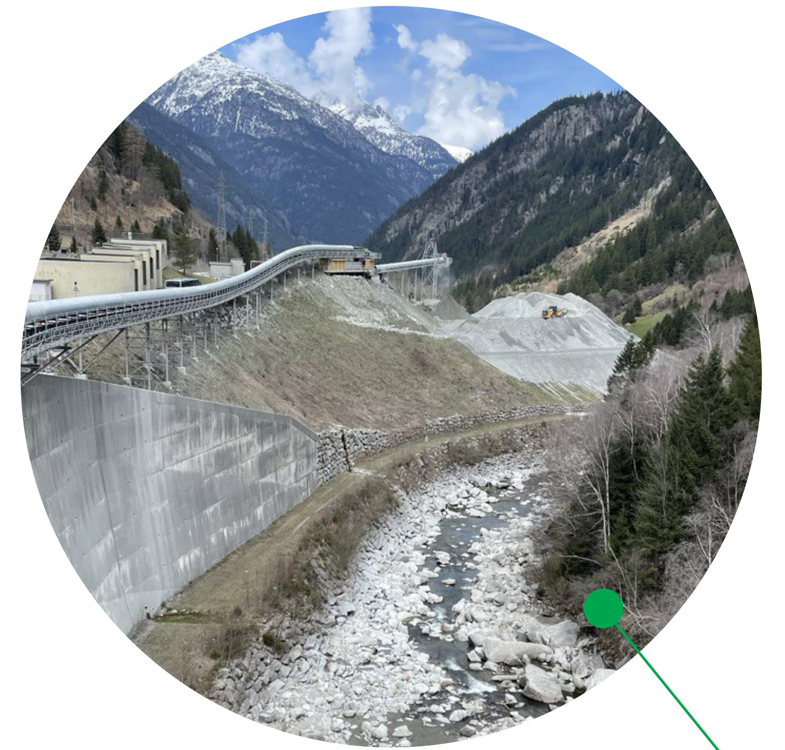
The view on the river by the construction site and landfill
