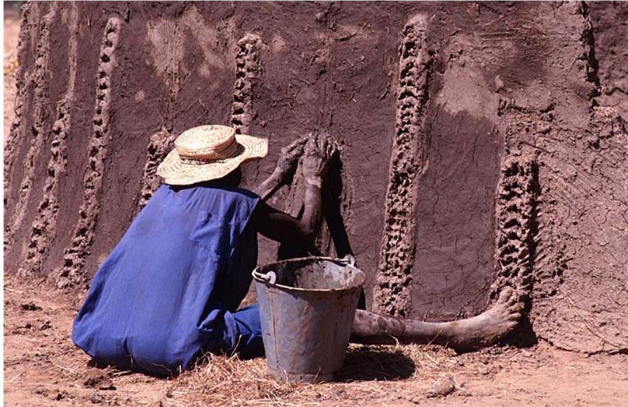
Photo of Musgum mud hut (Tolek) repair, Cameroon. Source: Vernacular Architecture Archive / Wikimedia Commons.
