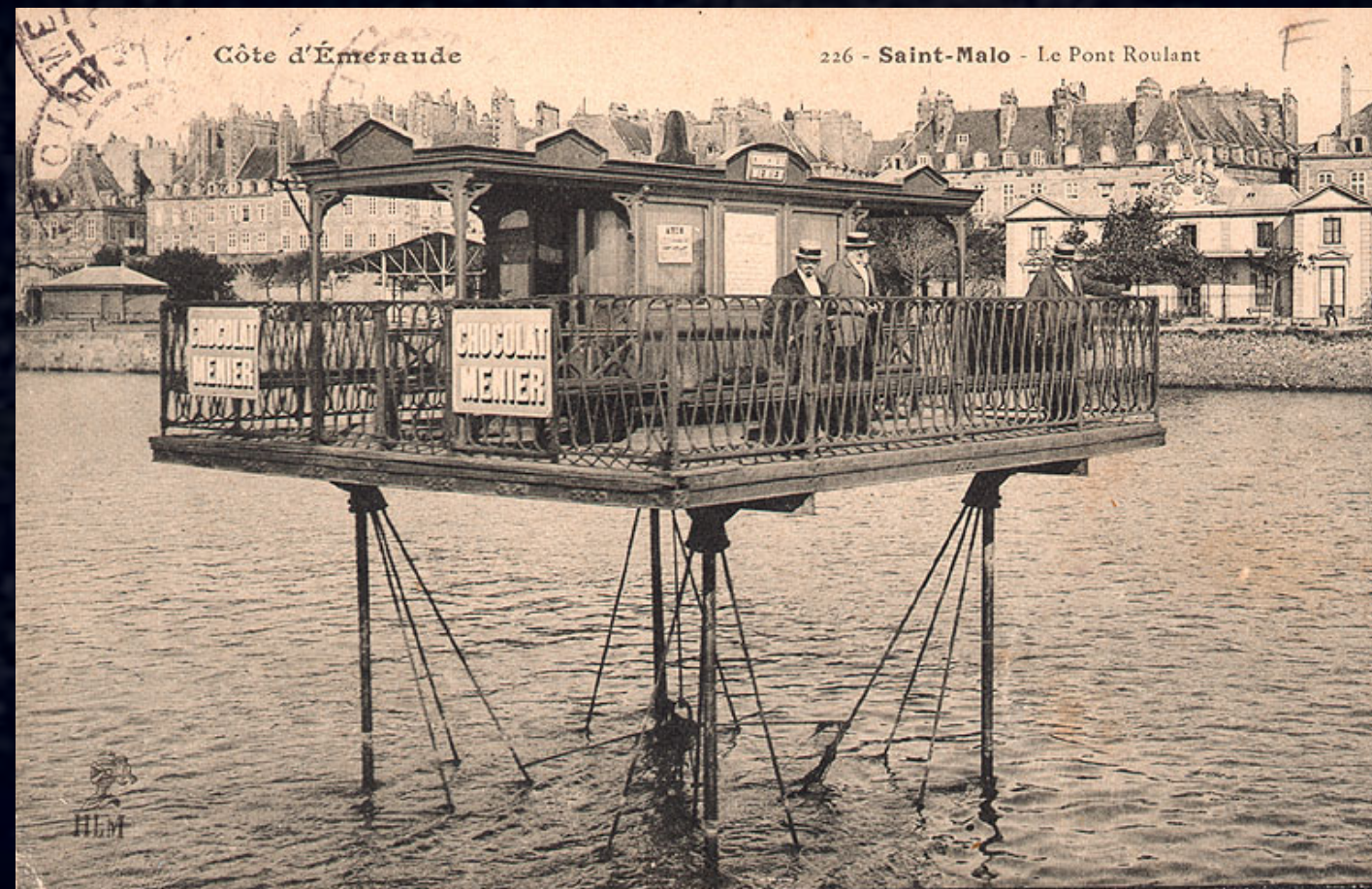
The historic Pont roulant de Saint-Malo (the Saint-Malo rolling bridge), an unusual tide-dependent vehicle that connected Saint-Malo and Saint-Servan in France, 1873-1923
