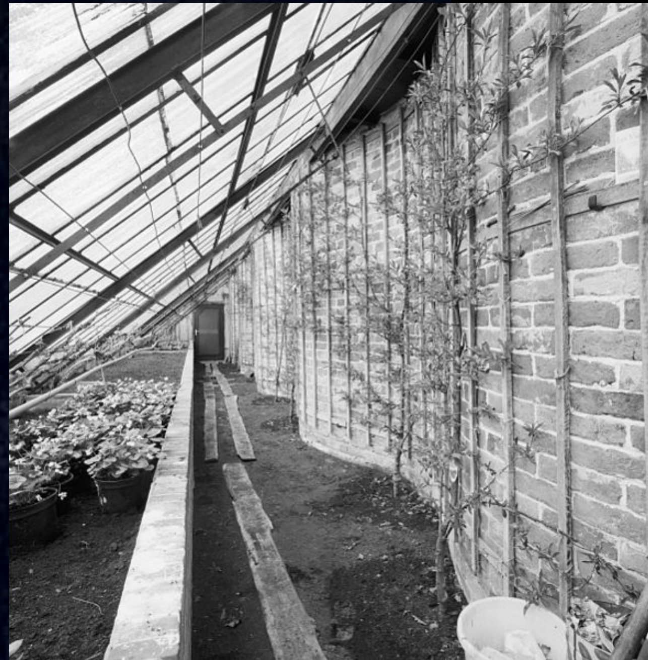
Greenhouse built against a serpentine fruit wall.
