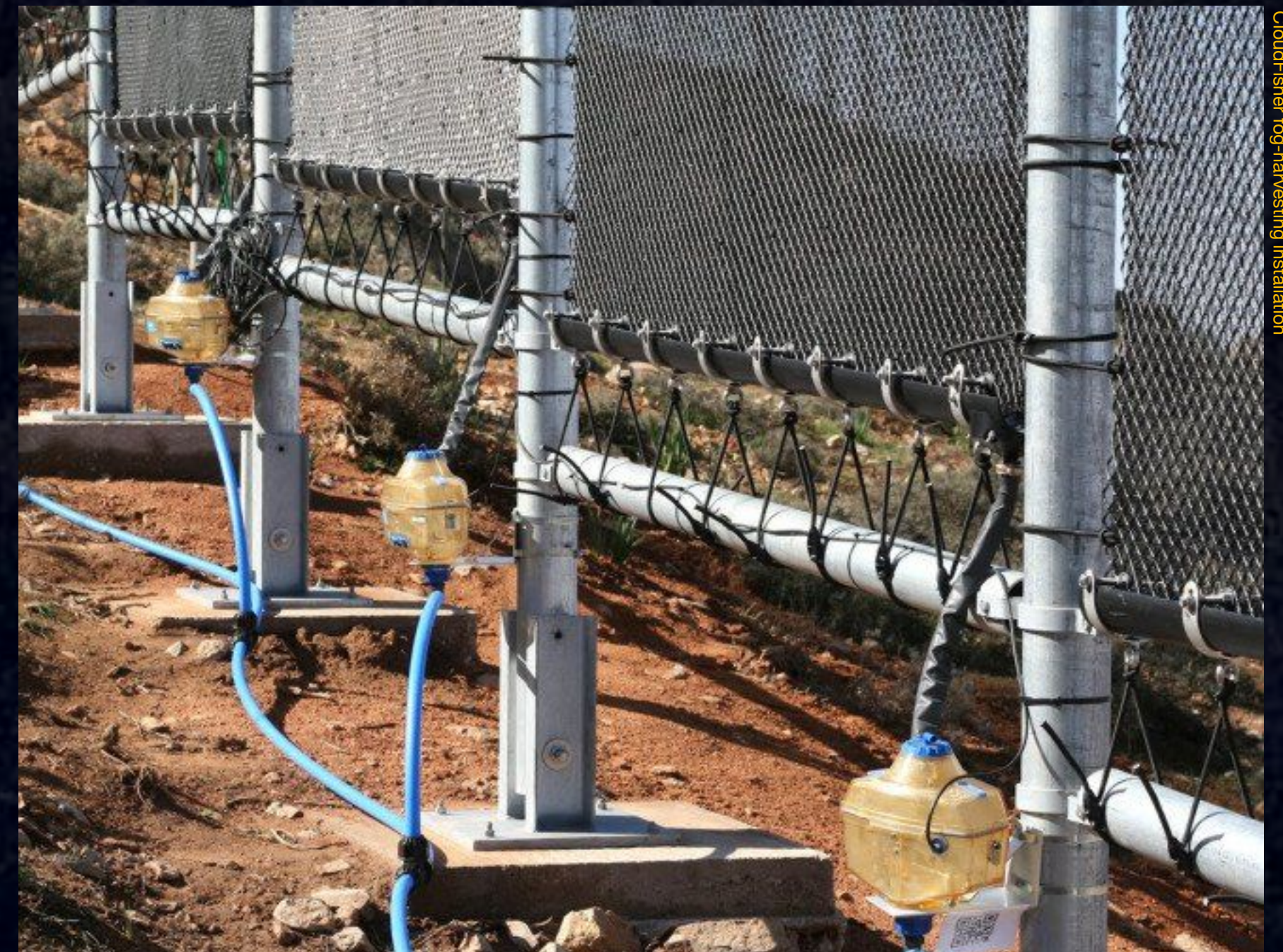
CloudFisher fog-harvesting installation
