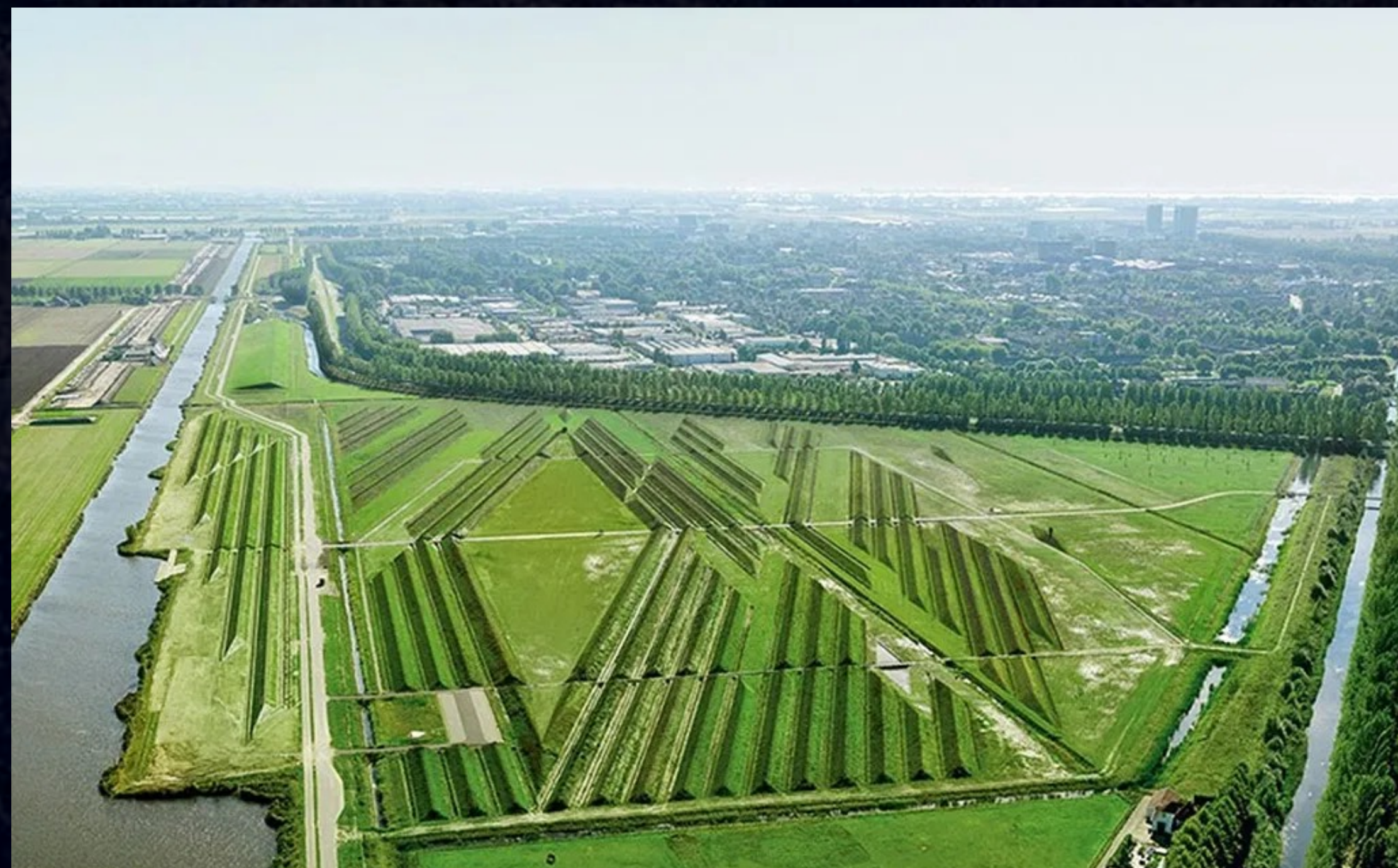
Sound Deflection Installation, Buitenschot Land Art Park L, Paul de Kort and H+N+S Landscape Architects, | Amsterdam Schiphol Airport,
