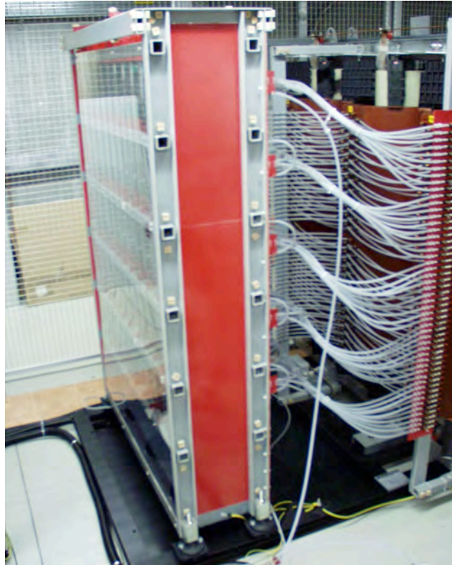
Fig. 3.6.3 BPS equipment installed inside the HV zone in the CRPP buildings. In front, the frame with the 50 power modules grouped in 5 rows and connected to the HV transformer behind.
