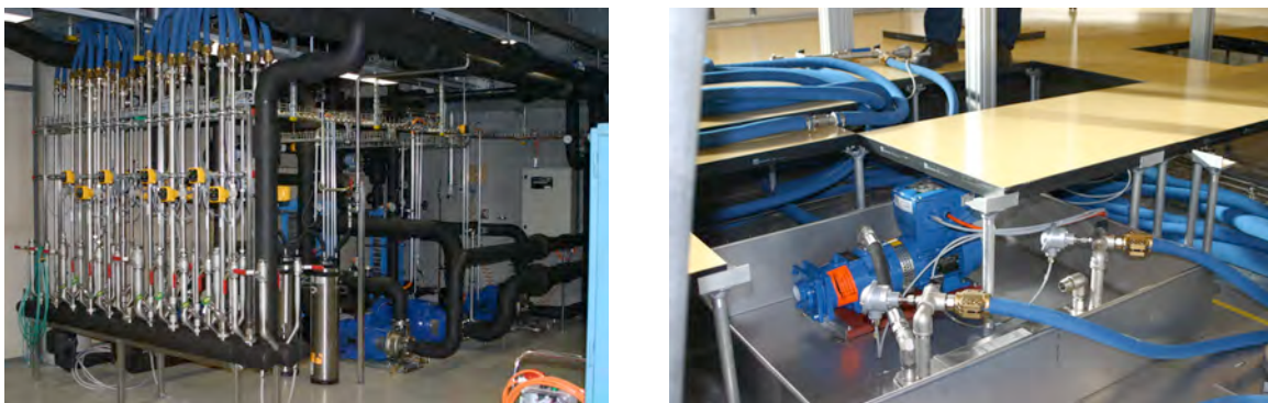
Fig. 3.6.7 Left: Distribution for the auxiliaries and pumps of the three circuits in the background. Right: Oil pump and heat exchanger ready to be connected to the gyrotron oil circuit.
