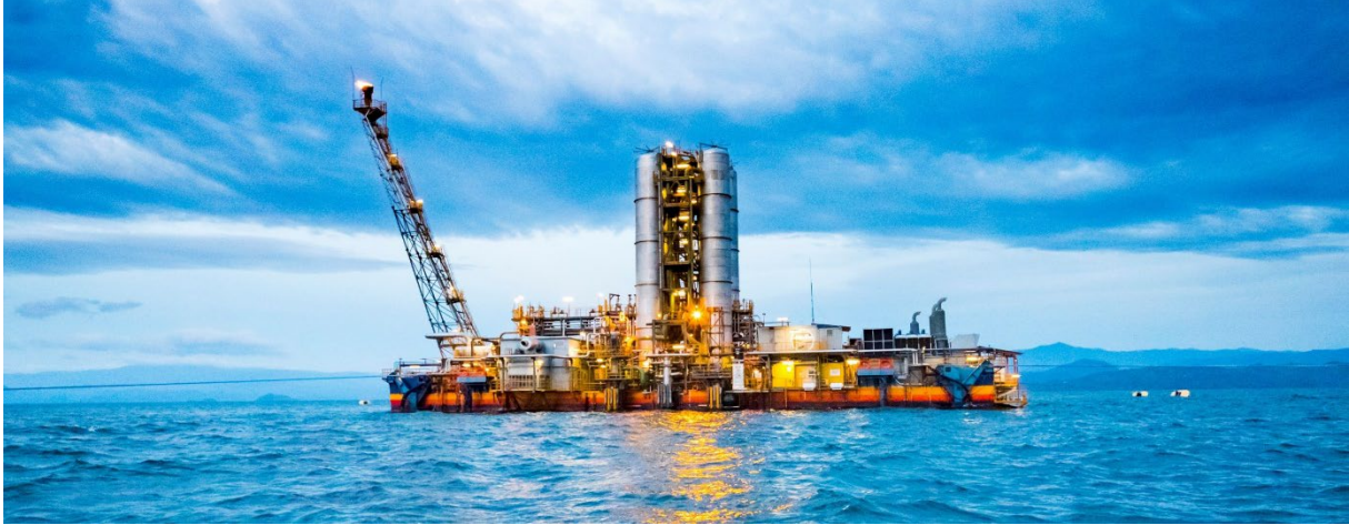
KivuWatt methane extraction plant ©ContourGlobal
