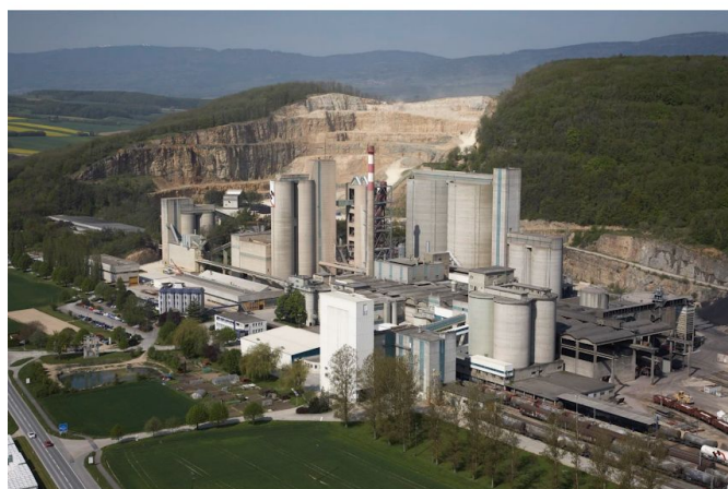
Cement production in Eclepens
