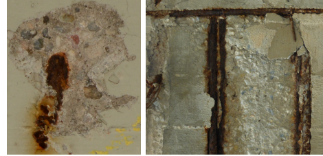
Figure 1: Two concrete image samples from CODEBRIM dataset, each have multiple overlapped defects. Left: Concrete with spallation, exposed bars and corrosion stain; Right: Concrete with spallation and exposed bars.
