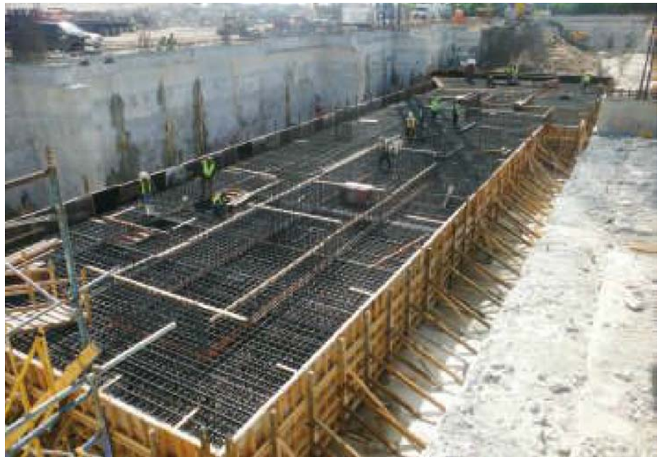
Tower construction of Oceana showing excavation
