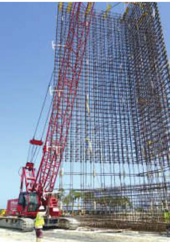
Slurry wall reinforcement at Oceana
