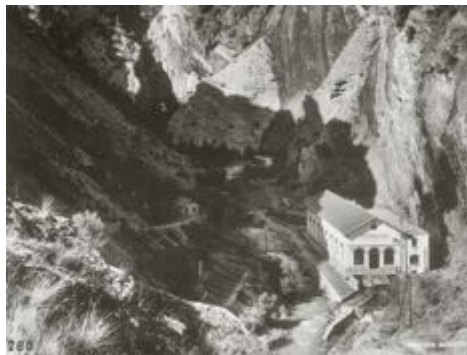
Hydroelectric plant Gampel 1898
