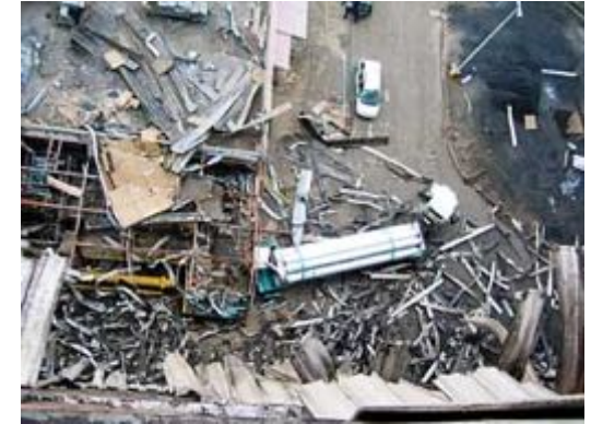
Tank explosion Muskingum River Power Plant's , USA, 8.1. 2007
