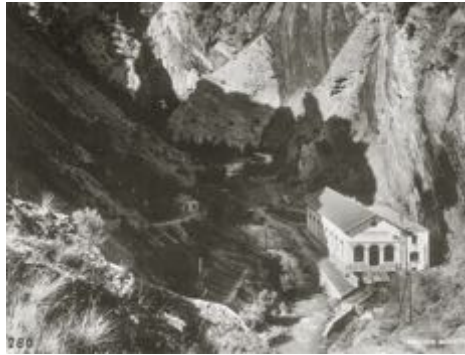
Hydroelectric plant Gampel 1898
