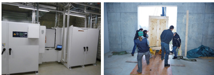
Fig. 4: Delivery and installation of the electrolyzers
