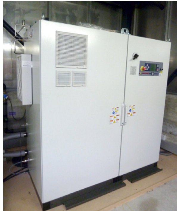
Fig. 2: The Proton OnSite Electrolyser will convert electricity overproduction into hydrogen
