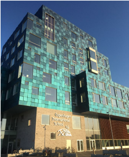
Copenhagen International School with solar cladding based on technology patented by LESO-PB
