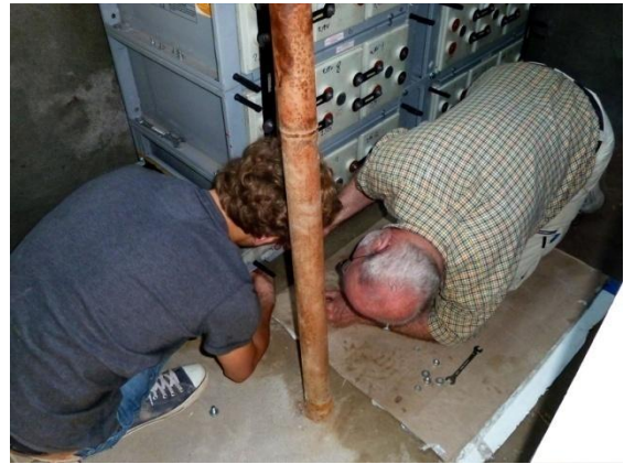
Figure 32: Me and Henri connecting the battery cells, 9 th of October 2011 (4).
