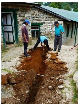
Figure 27: Two locals and Phurba digging a trench for the electric cables, 8 th of October 2011 (4).
