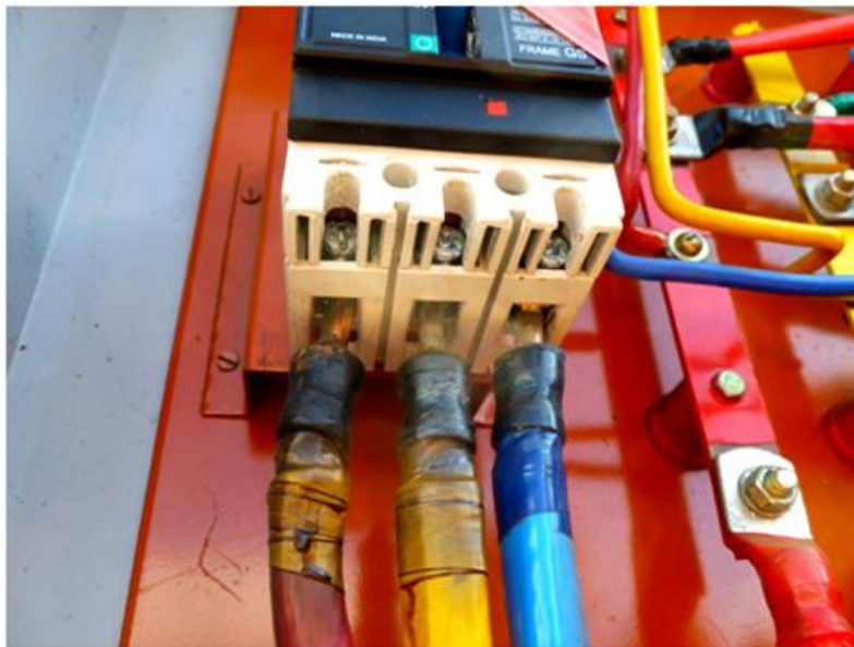
Figure 5: Detailed view of a distribution cubicle, the red cable was burned (9).
