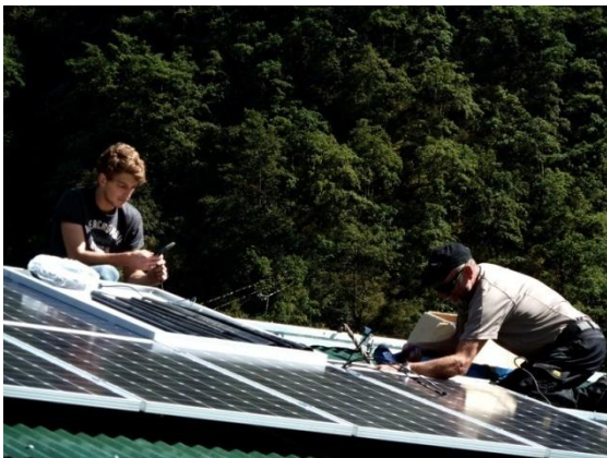
Figure 35: Me and Bernard connecting the solar panels, 11 th of October 2011 (4).
