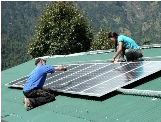
Figure 33: Bernard and Purnima mounting the solar panels on a rack, 10 th of October 2011 (4).
