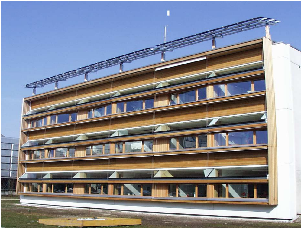
Figure 1-1. View of the south facade and the PV installation of the LESO building
