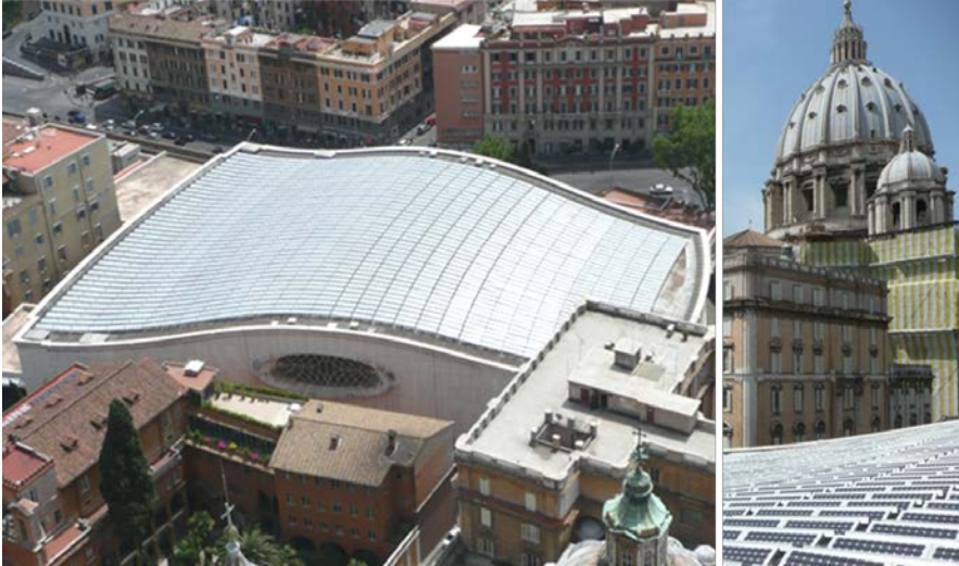
PV system on the roof of Aula Pierluigi Nervi Vatican City.
