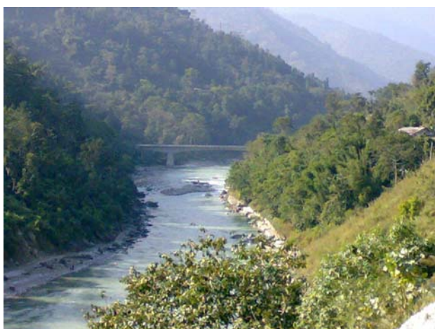
Fig. 1: Upstream view of the Teesta River at the future dam site
