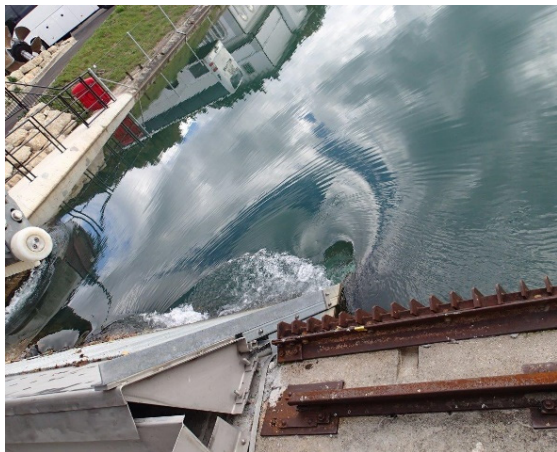
Figure 1: Grande vortex de grande surface à l'entrée de la turbine M5 / Large surface vortex at the turbine M5 inlet opening.
