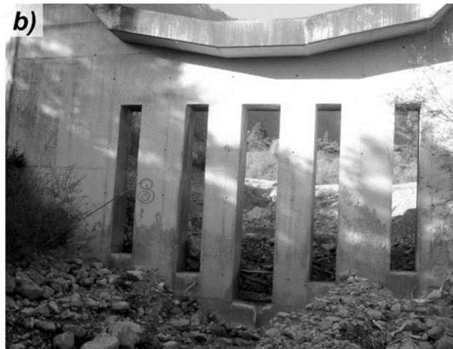
Figure 1: Illustration of two basic types an open check dam, a) an open-gap crested check dam [Riddes, VS] and b) closed crest type check dam [Manival, France].
