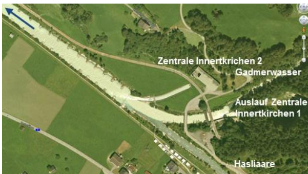
Figure 1 : Restitution existantes des centrales Innertkirchen 1 et 2. / Existing restitution of the power plants Innertkirchen 1 and 2.
