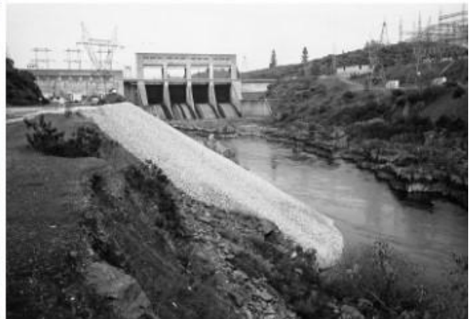
Figure 1 : Examples of replenishment of sediments: (left) replenishment in Aargau Canton, Switzerland, between 2009-2012; (right) gravel replenishment to the Sacramento River below Keswick dam.
