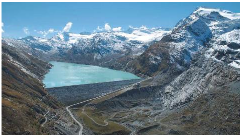
Figure 1 : Barrage de Mattmark (source: Swiss Committee on Dams).
