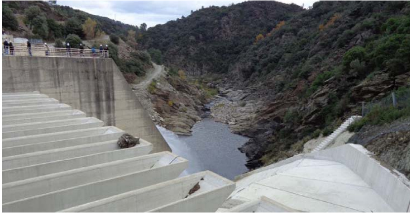
Malarce Dam with PKW
