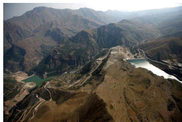
Figure 2: Siah-Bishe pumped-storage dam and power plant, Iran
