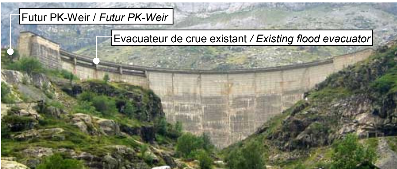
Figure 1: Figure 1: Vue de la face aval du barrage existant des Gloriettes /View of the downstream face of the existing dam
