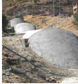
Figure 2: View looking upstream showing the stair-step structure.
