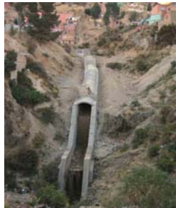
Figure 1: General view of the sewer pipeline
