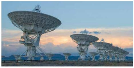
Figure 50 The Very Large Array (VLA) is a collection of 27 radio antennas located at the NRAO site in Socorro, New Mexico. Each antenna in the array measures 25 meters (82 feet) in diameter and weighs about 230 tons. Credit Alex Savello / National Radio Astronomy Observatory
