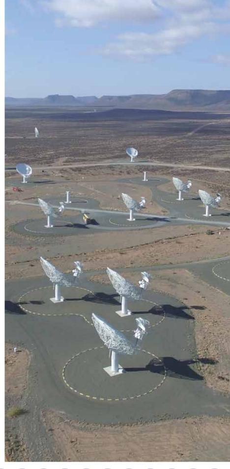
Figure 28 Aerial shot of the MeerKAT radio telescope before its launch in July 2018. These sunrise shots show the expanse of the telescope, which covers a baseline distance of 8 km.Credit : South African Radio Astronomy Observatory (SARAO)
