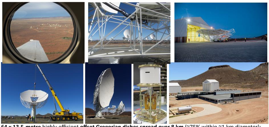
**64 x 13.5-metre** highly efficient **offset Gregorian dishes spread over 8 km** (~75% within ~1 km diameter); superb L-band receivers (**0.9–1.67 GHz**); also UHF (**0.58–1.0 GHz**) and S-band (**1.75–3.5 GHz** – by MPIfR)
