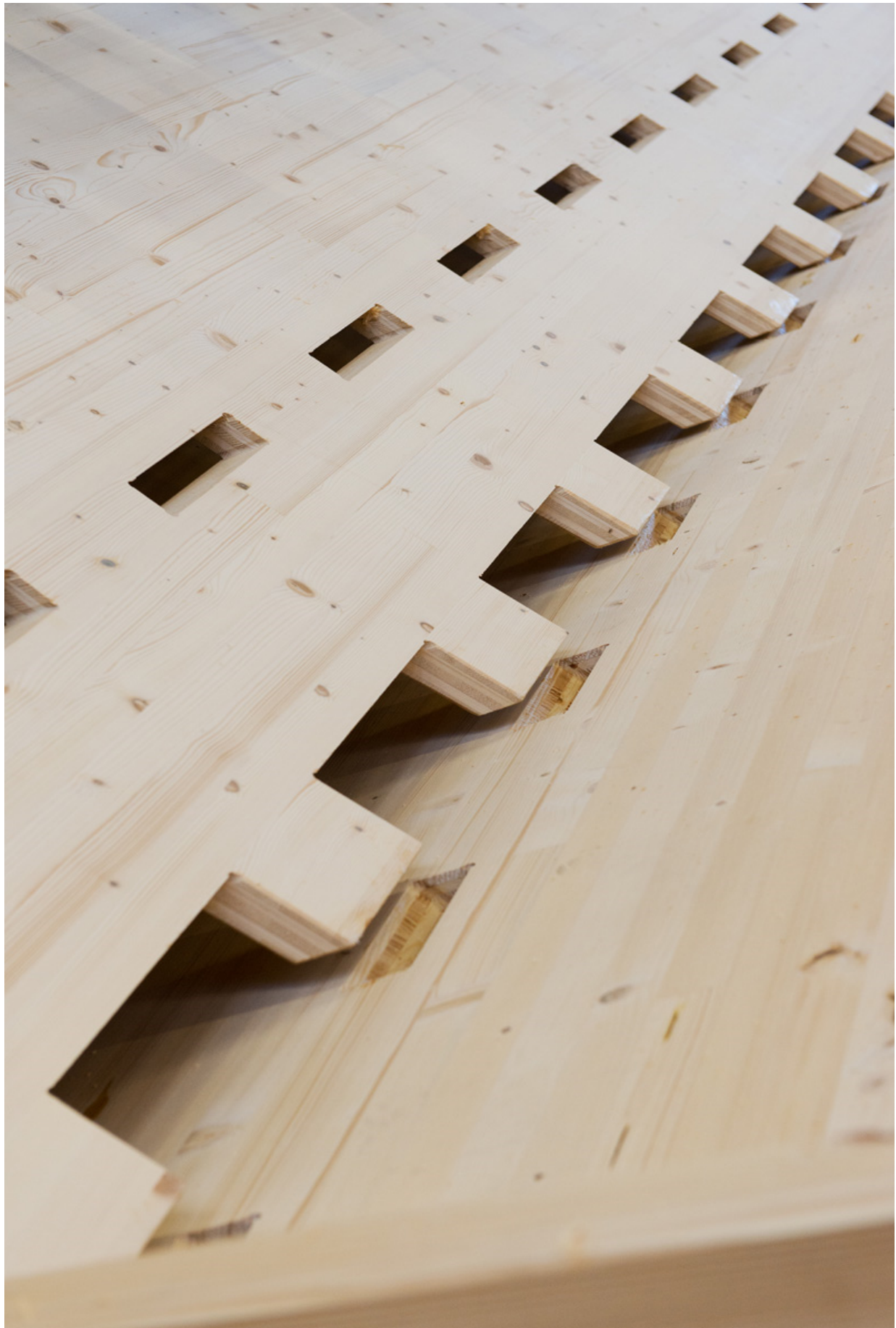
Figure 5. Assembly of the integral joints (credits: I. Kramer)
