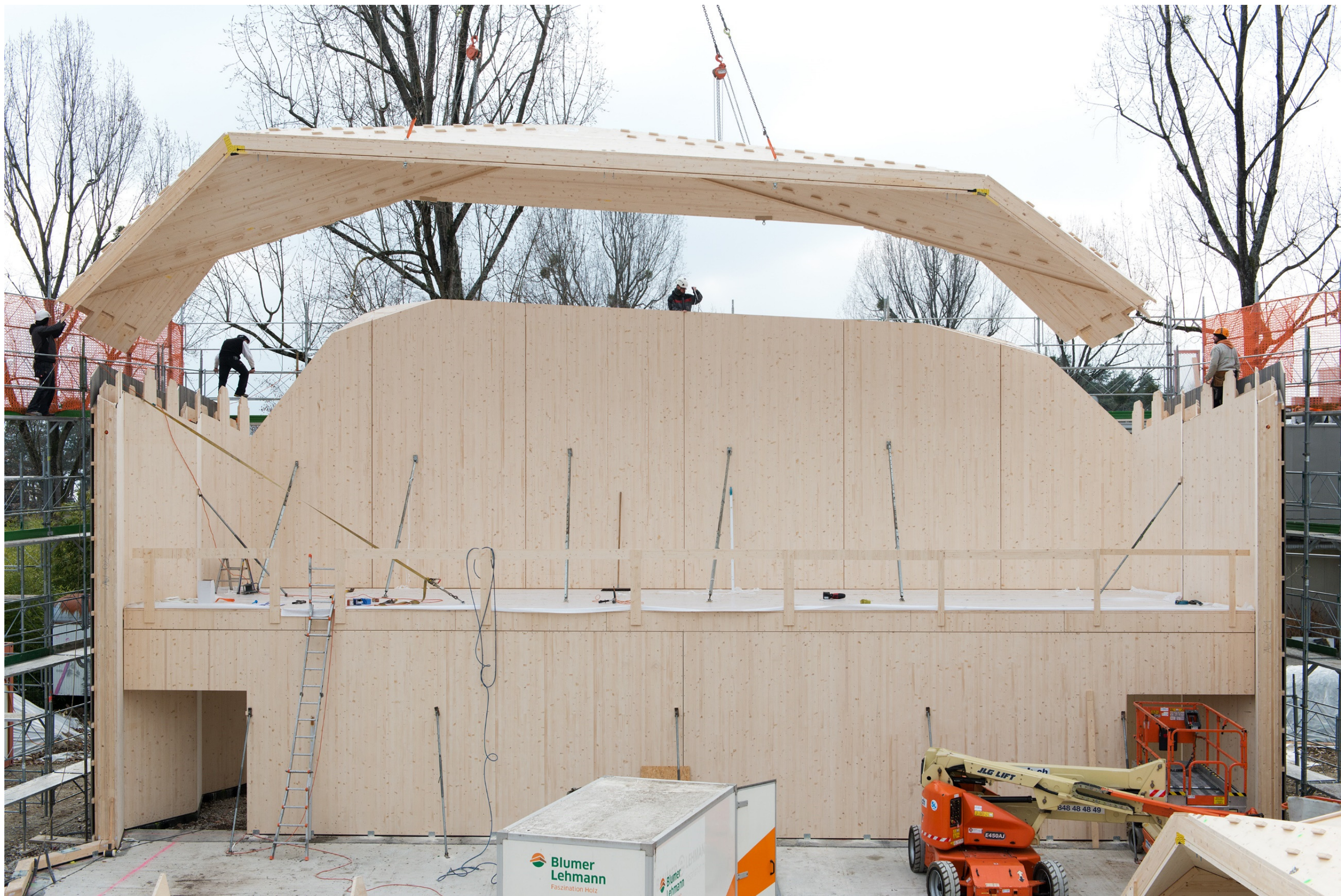
Figure 1. Construction of the timber pavilion of the Vidy-Lausanne theatre: assembly of the first roof segment (18m span) (credits: I. Kramer)
