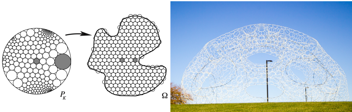
Figure 1: Left: Discrete Riemann mapping with circle packing [4]. Right: Dome structure built with thousands of woven circles of composite fibre [1].
