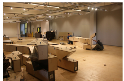
filename: 12_MJHL_construction_2.jpg © ALICE Studio EPFL + ECAL Lab
