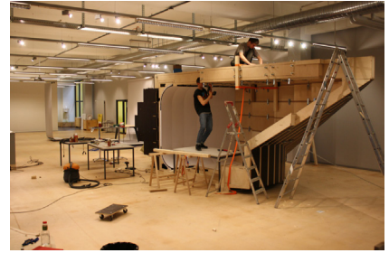
filename: 15_MJHL_construction_5.jpg © ALICE Studio EPFL + ECAL Lab
