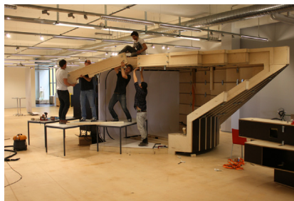
filename: 17_MJHL_construction_7.jpg © ALICE Studio EPFL + ECAL Lab
