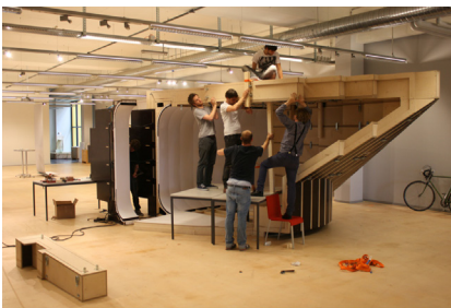
filename: 16_MJHL_construction_6.jpg © ALICE Studio EPFL + ECAL Lab
