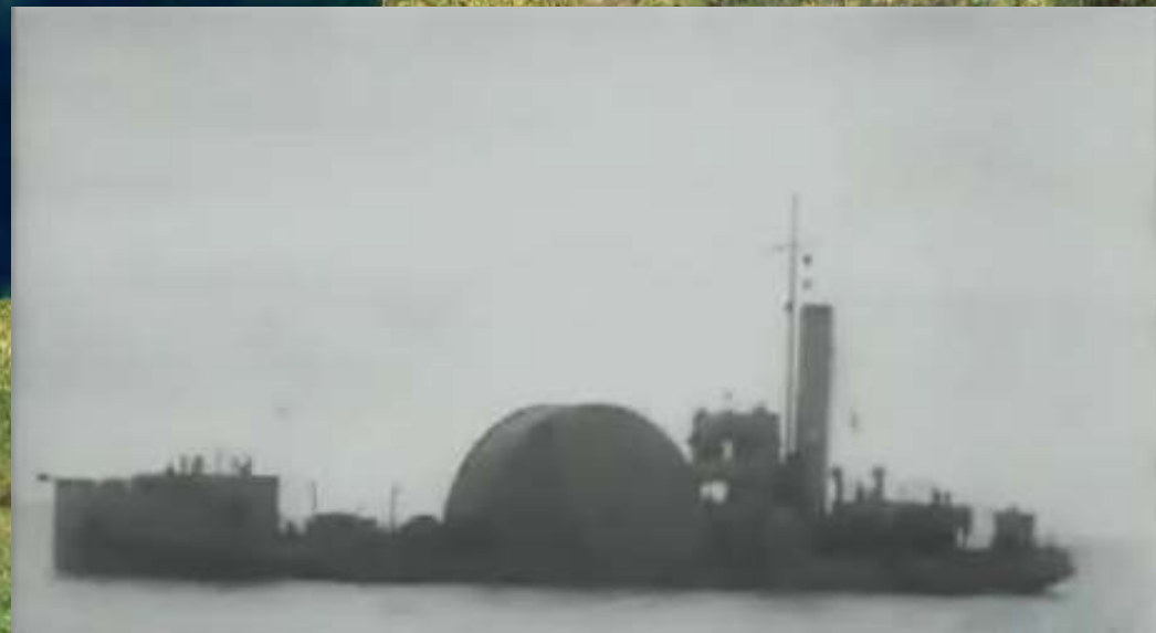
PipeLine Under The Ocean (PLUTO), 1944
