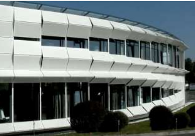
Kiefer Technic Showroom
