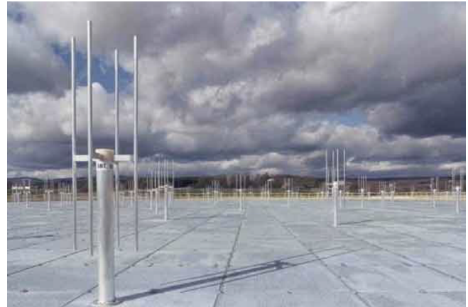
Fig. 4. Reception site for the GRAVES system. There are 100 antennas dispatch in a circle area.
